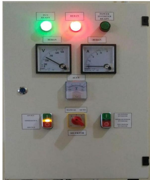
Figure 2. Automatic transfer switch operation on PLN electricity and power inverters
