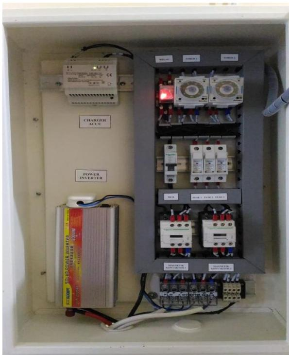
Figure 3. The automatic transfer switch panel device appears inside the panel
