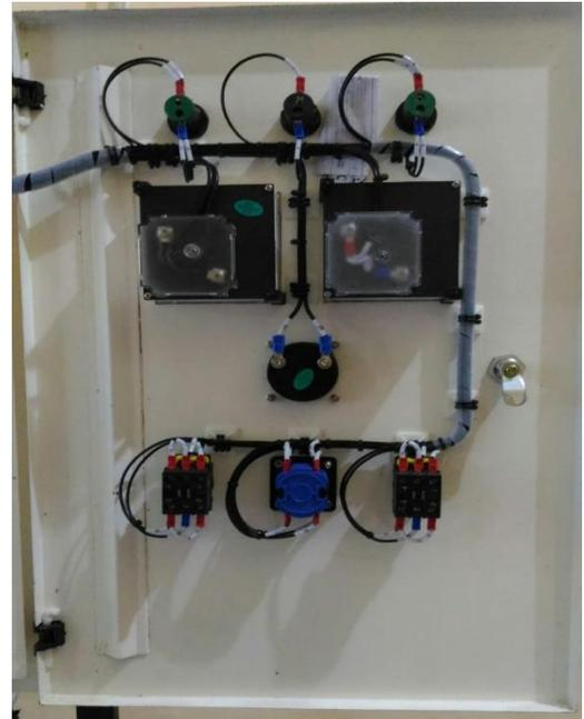
Figure 4. The inside door panel automatic transfer switch appears on the door panel
