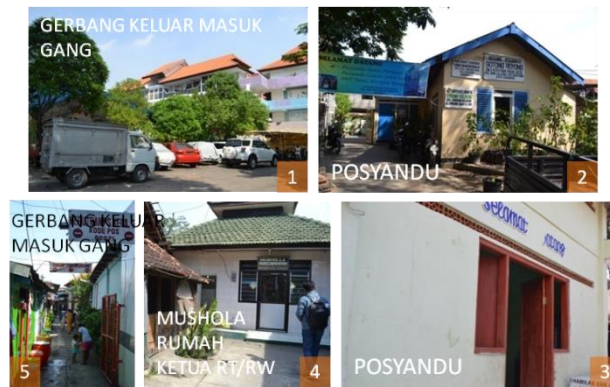
Figure 11 Buildings and physical conditions at the study location
